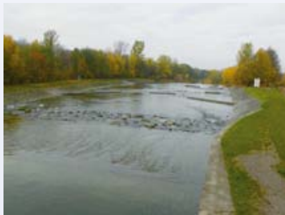
Stone-wire pylons in the Moravka river.
