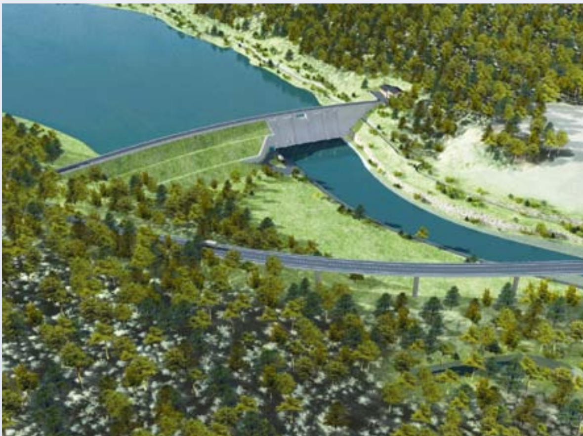
Vizualization regarding one of possible options related to the dam of the water reservoir Nové Heřminovy being prepared there.
