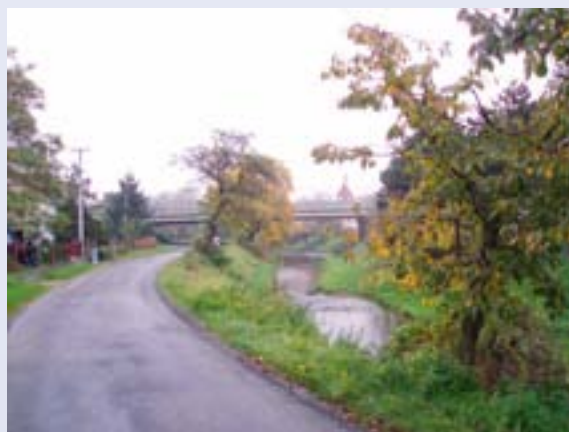
Current condition of the water course Ondřejnice. The project „Regulation of the Ondřejnice river, Stará Ves nad Ondřejnicí” will provide protection of the village against 20-year water.
