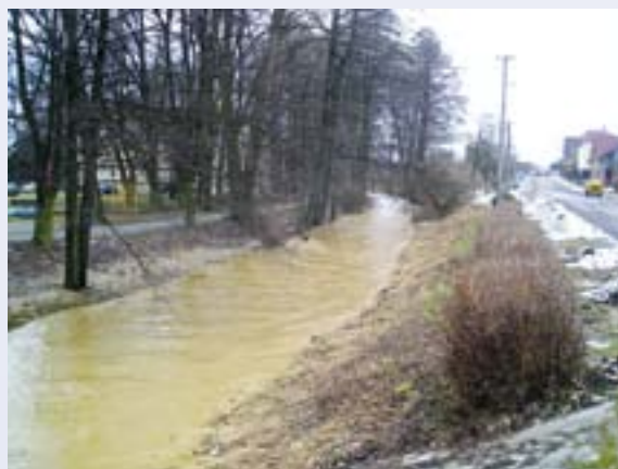
Floods on the Porubka river in Ostrava-Svinov threaten buildings and technical infrastructure. The project „Regulation of the Porubka river, Ostrava-Svinov” will provide protection against floods up to Q_{20} flow rate.
